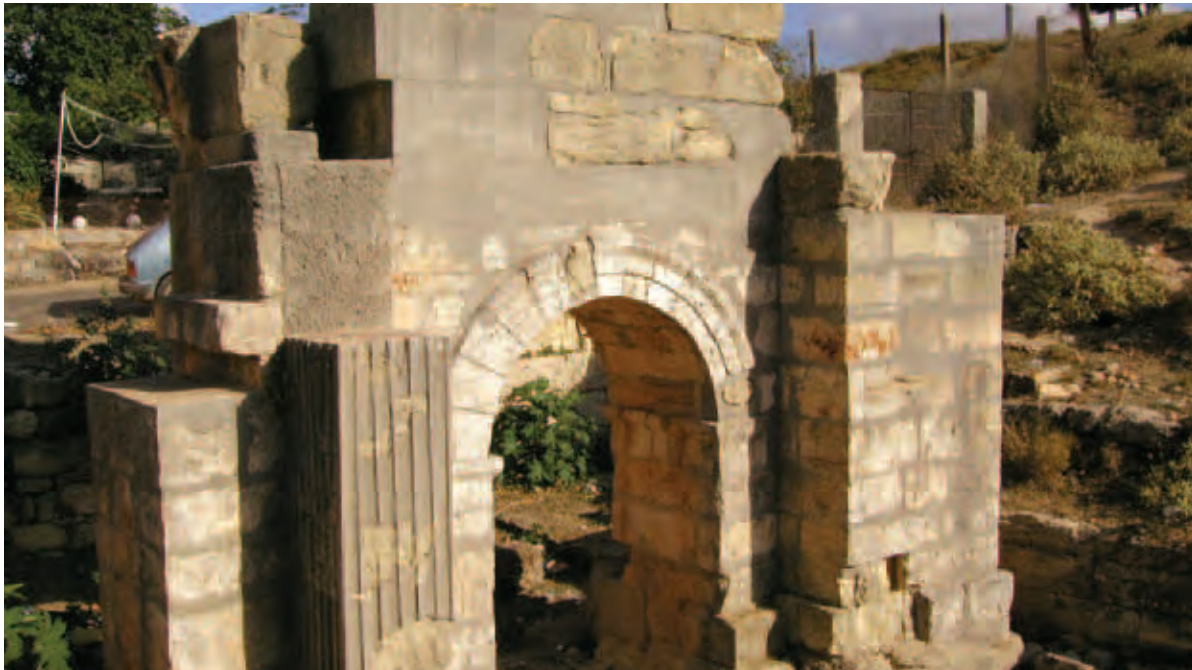
In Cyrene, Libya, a UNESCO World Heritage Site, Portland cement and rebar is used to patch together ancient monuments even today. Inappropriate reconstructions and unauthentic restorations for tourism are one of the most severe causes of loss and destruction to global heritage sites. Photo: GHF
