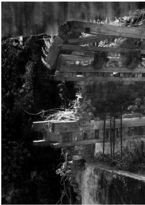
Fig. 9 and 10 Views of ruins of a house in the walled city of Ahmedabad, showing a form of timber lacing similar to that found in taq construction in Kashmir. In the partially dismantled building, the construction with runner beams tied together with cross-timbers pegged to the beams is visible (photographs © Randolph Langenbach)
