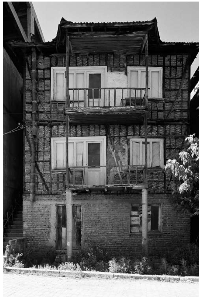
Fig. 5 This three story house in Gölcük located less than one km from the fault was undamaged by the 1999 earthquake, while a number of reinforced concrete buildings on the adjacent blocks collapsed (photograph © Randolph Langenbach)
