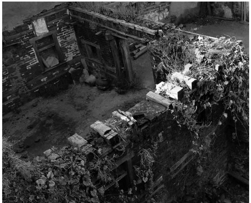
Fig. 9 and 10 Views of ruins of a house in the walled city of Ahmedabad, showing a form of timber lacing similar to that found in taq construction in Kashmir. In the partially dismantled building, the construction with runner beams tied together with cross-timbers pegged to the beams is visible (photographs © Randolph Langenbach)
