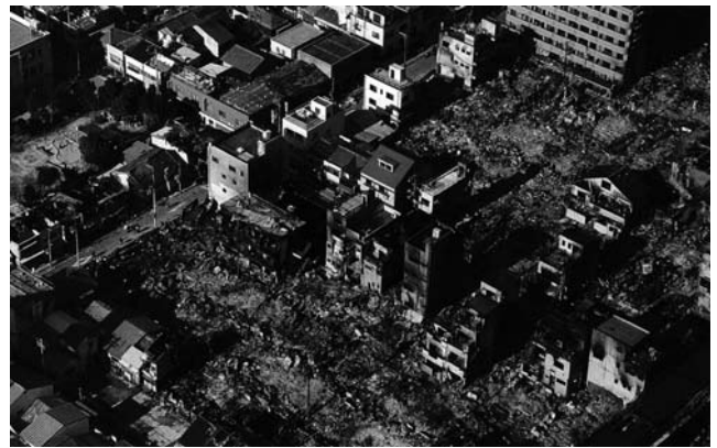
Fig. 2 Earthquake damage in Kobe, Japan, 1995. The fire department had to give up entire blocks and retreat to fire-breaks (in this photo a broad street) in order to fight the flames
