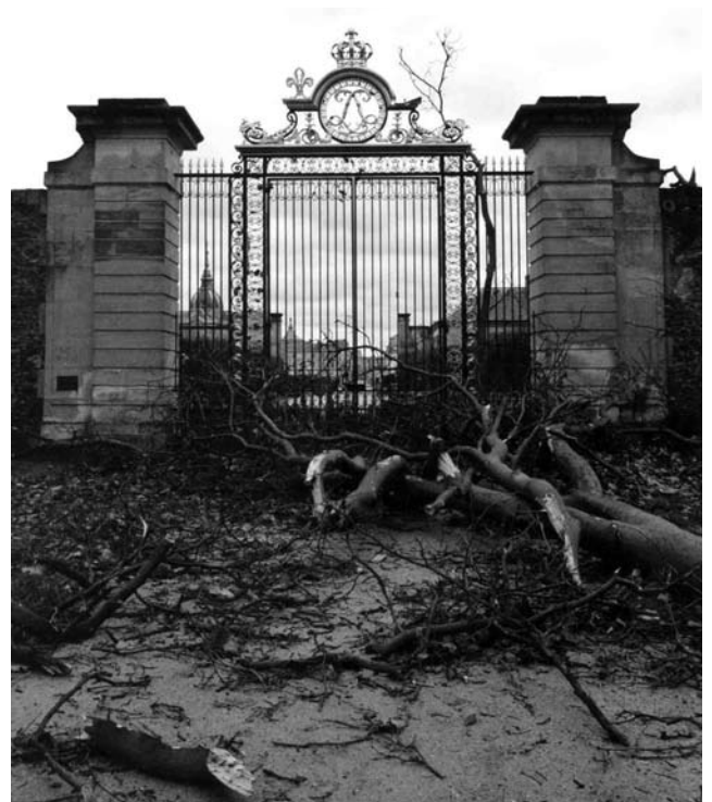
Fig. 8 Versailles, Swiss Gate with storm damage
