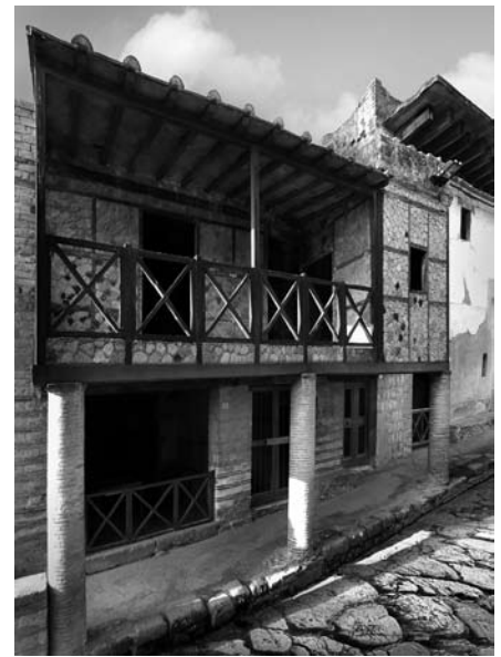
Fig. 8 The Craticii House at Herculaneum, 2003 (photograph © Randolph Langenbach)
