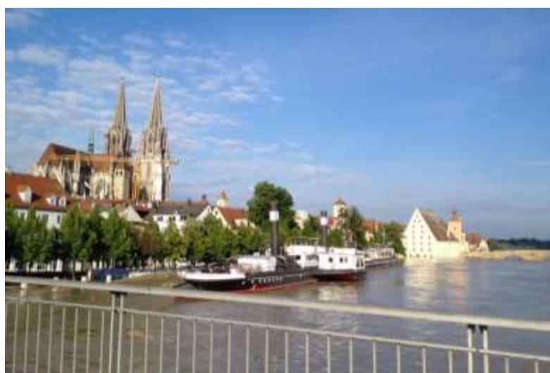
Figure 3. Flooding is a serious threat to the 'World Heritage Site Old Town of Regensburg with Stadthof' (Photo: Susanne Hauer)
