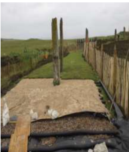
Figure 7. Engineered footpaths: pipe laid across width of path to drain into external ditch (Credit: HES)
