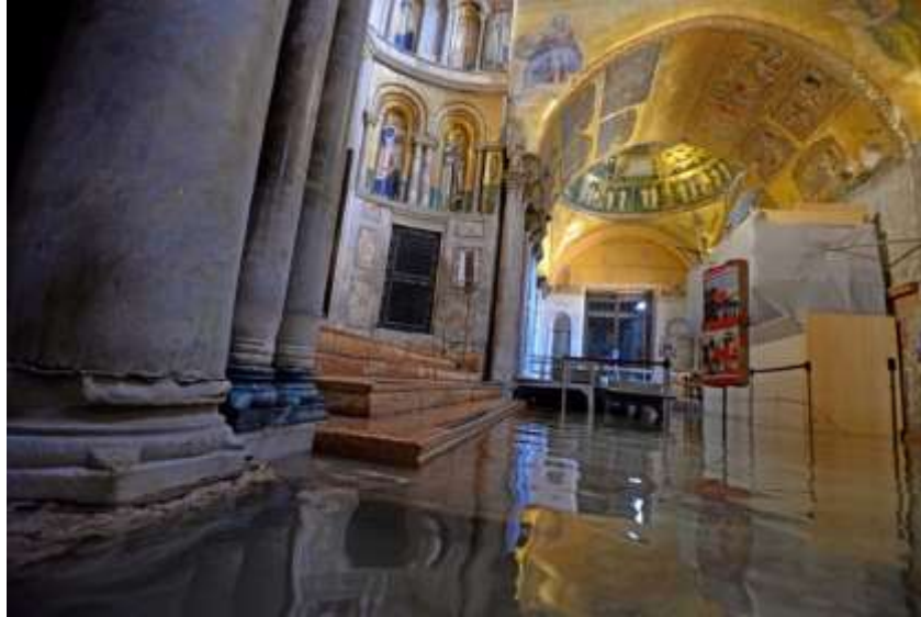
Figure 12. The narthex (atrium) of the St Mark's Basilica flooded. On the night of the 12 th November the level of the water overcame the four visible steps, flooding also the main Basilica's floors
