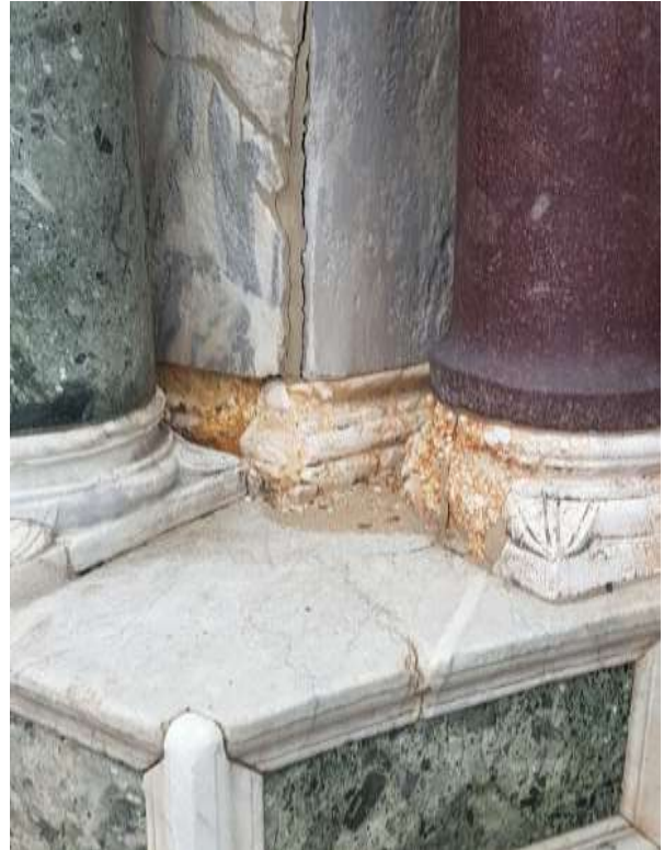
Figure 10. The effects of increased pressure by salty water, air pollution (SOx), and more intense use on the basis of two marbles columns of the St Mark's Basilica front
