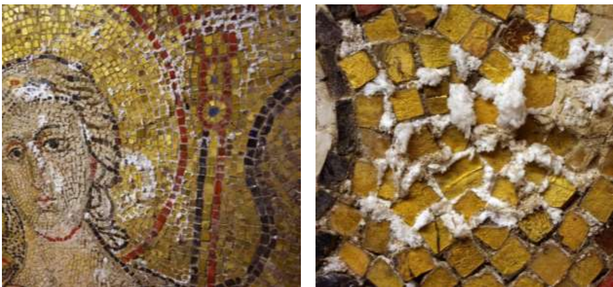
Figure 9. The salty water infiltrates by capillarity the tiles of this mosaic located 12 m off the pavement
