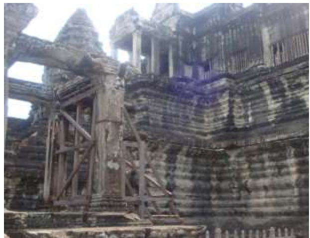
Figure 15. Two temples in Angkor that required to be supported because of land subsidence (Photos: Fulong Chen)
