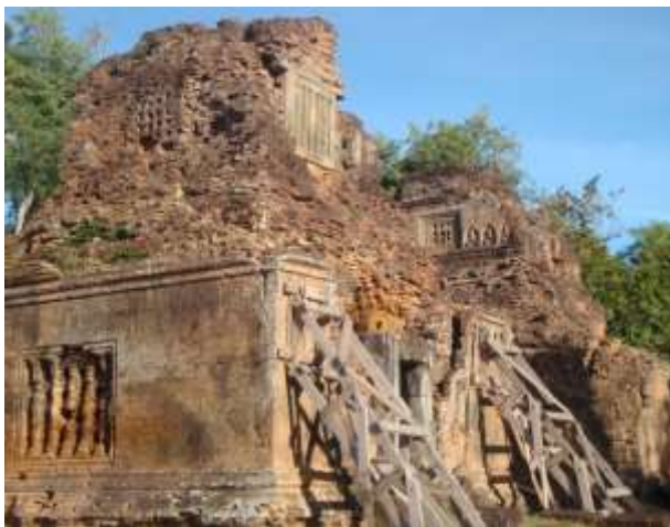
Figure 15. Two temples in Angkor that required to be supported because of land subsidence (Photos: Fulong Chen)
