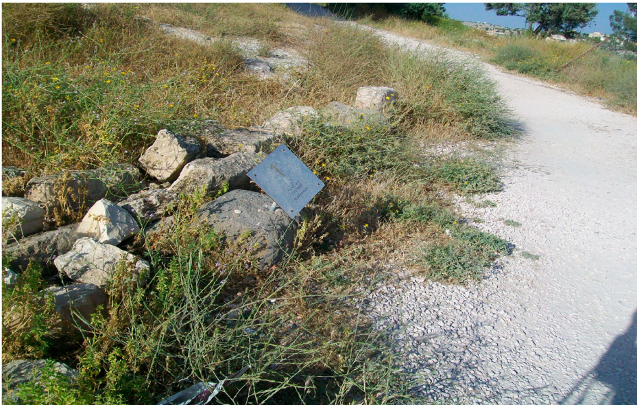
Figure 7. Inadequate design with accessibility needs. Source: Author.
