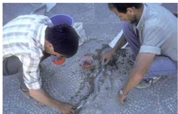
Fig. 9. Filling of a fracture in a mosaic with lime mortar
