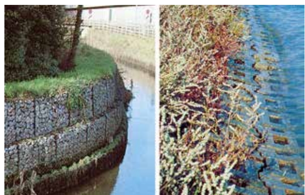
Fig. 7. Protection of an embankment with gabions (Maccaferri)
