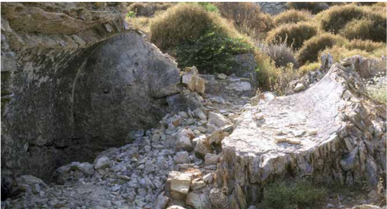
Fig. 4. Erosion of a hill slope and rainwater runoff is a common cause of the destruction of archaeological deposits and structures, such as the collapse of this Roman vaulted chamber in southern Turkey
