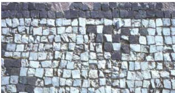
Fig. 10. A mosaic re-laid in a good lime mortar base, but with fractured tesserae still subject to environmental erosion
