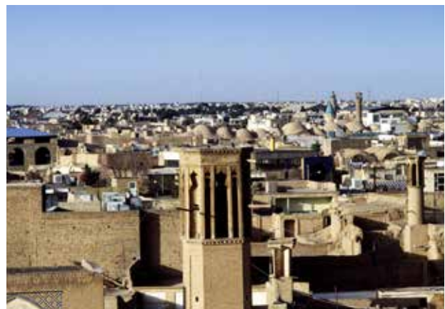
Fig. 5. Kashan. The historic city of Kashan, Iran, has retained much of its historic integrity, particularly that of its building fabric, and its wind-tower-based traditional ventilation system. In recent years, housing complexes have been rehabilitated as hotels. However, many of its fragile mud brick buildings risk decay and even collapse if not properly used and regularly maintained.
