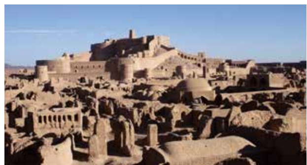
Fig. 4. Bam. The ancient citadel of Bam, Iran, developed particularly in the early Islamic period. Since the earthquake of 2003, it has been subject to an international conservation project. The citadel has been recognized as part of a vast cultural landscape, where life is shaped by a traditional water management system. The site was inscribed on the World Heritage List in 2004.
