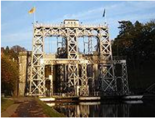
Lift No. 2, The four lifts on the Canal du Centre (Photo use licensed under Wikimedia commons)
